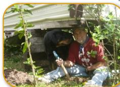
Bill, being supervised by Shaka, is removing the rotten posts that were holding up one of the dorm buildings. Once removed, we will pour in a concrete foundation and put on a new hardwood post to support the building.
